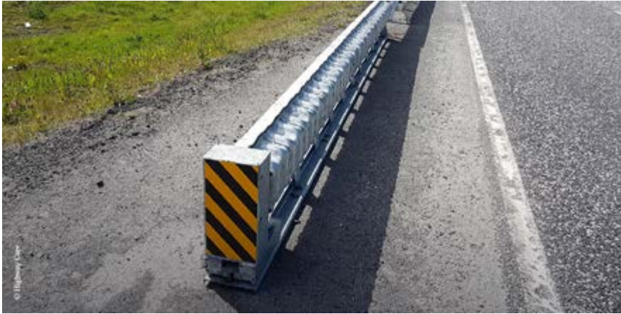
Figure 3 — Energy-absorbing barrier terminal (photo: courtesy of Highway
