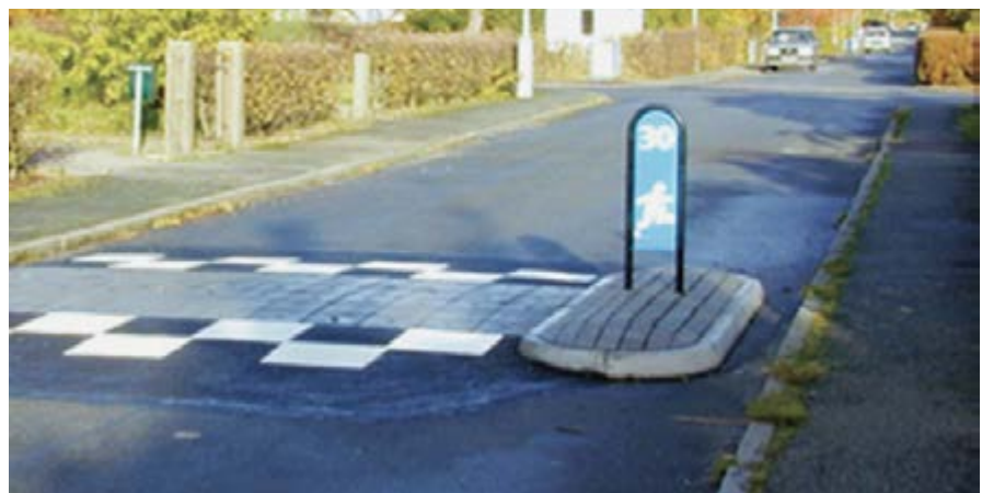
Figure 4 — speed hump on a local street in Gothenberg, Sweden
