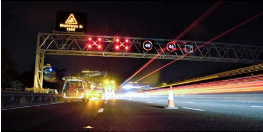
Figure 7 — Automatic lane closure and enforcement system, United Kingdom (photo: courtesy of Redflex)
