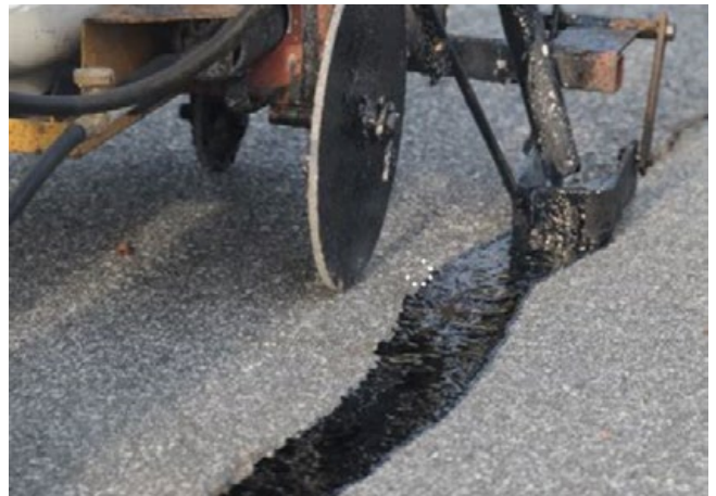
Application of a proprietary binder bandage crack seal Photographer unknown
