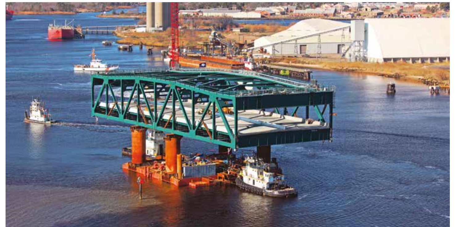
Gilmerton Bridge Chesapeake, Virginia Construction Engineering and Inspection
