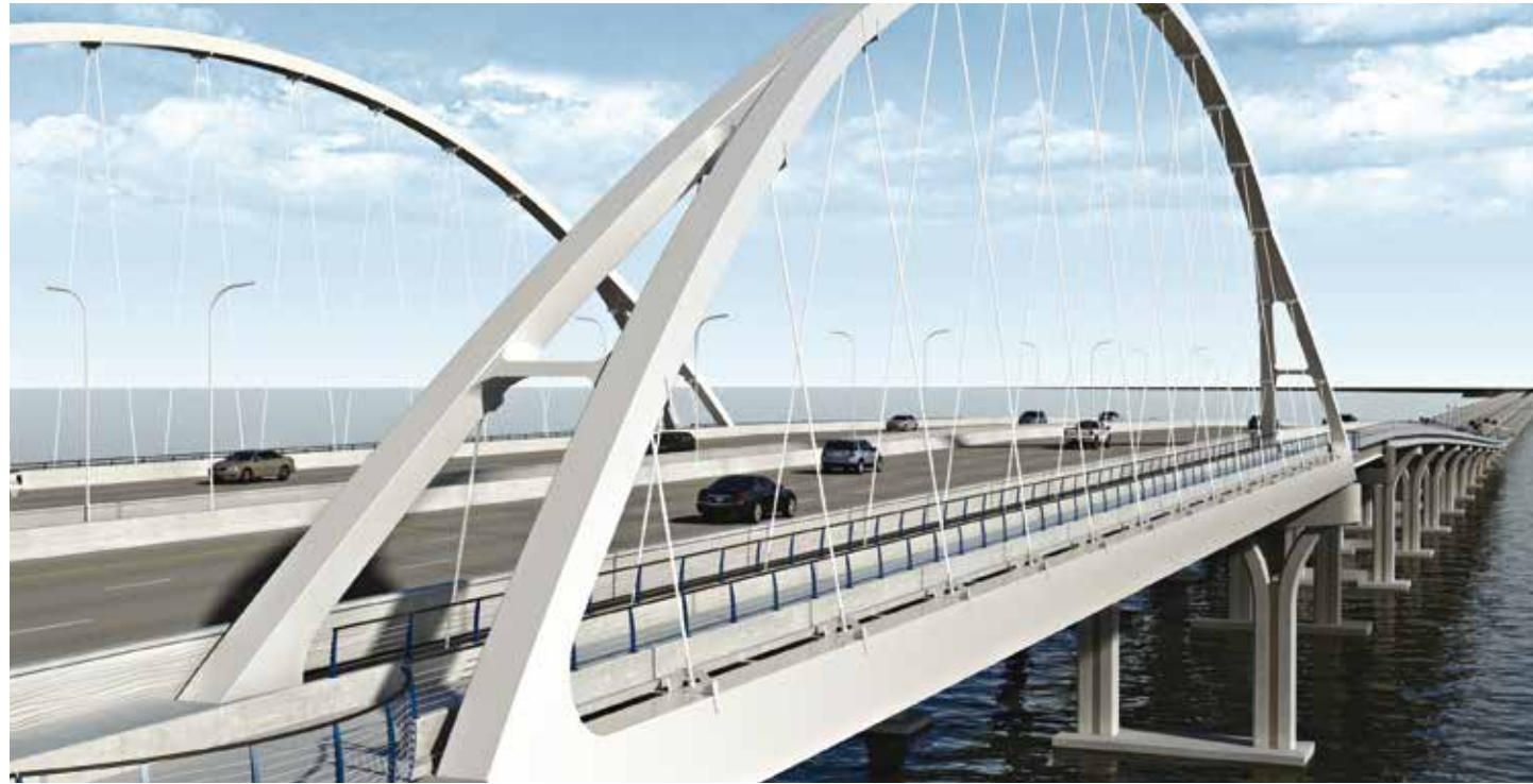
Pensacola Bay Bridge Pensacola, Florida Design
