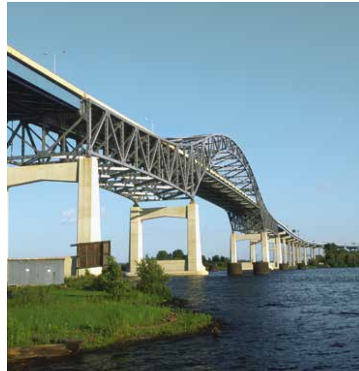
John A. Blatnik Bridge Duluth, Minnesota Inspections; Design; Asset Management
