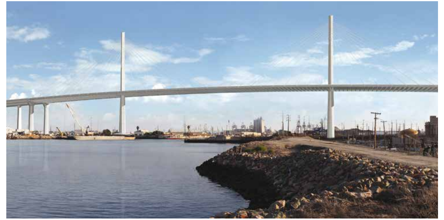
Gerald Desmond Bridge Long Beach, California Program and Construction Management
