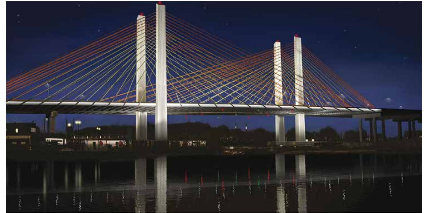
Kosciuszko Bridge New York, New York Planning; Design; Construction Services
