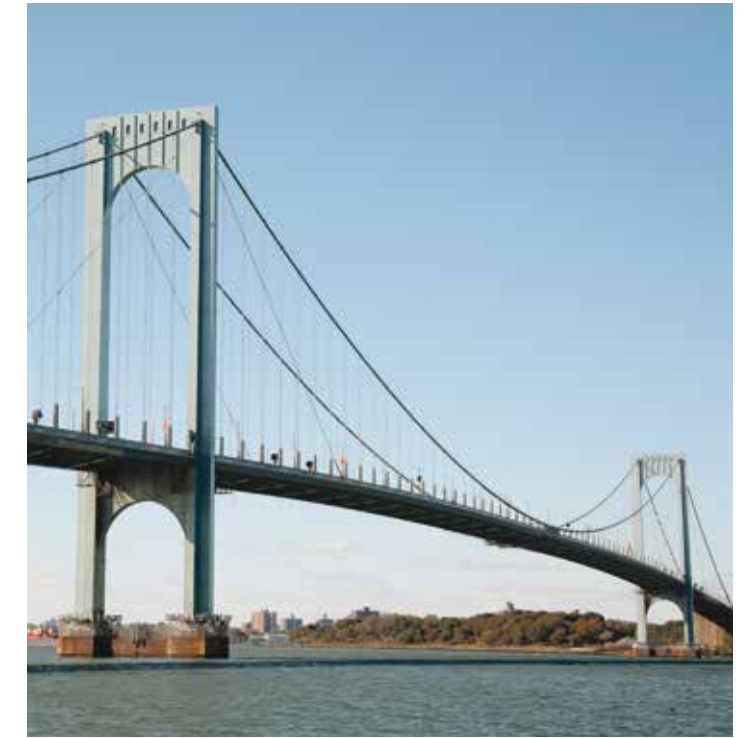
Bronx-Whitestone Bridge Bronx, New York Biennial and Special Inspections; Feasibility Study; Construction Management
