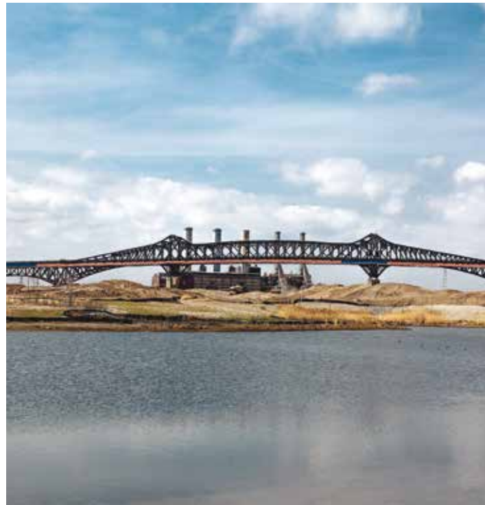
Pulaski Skyway Rehabilitation Jersey City, New Jersey Design
