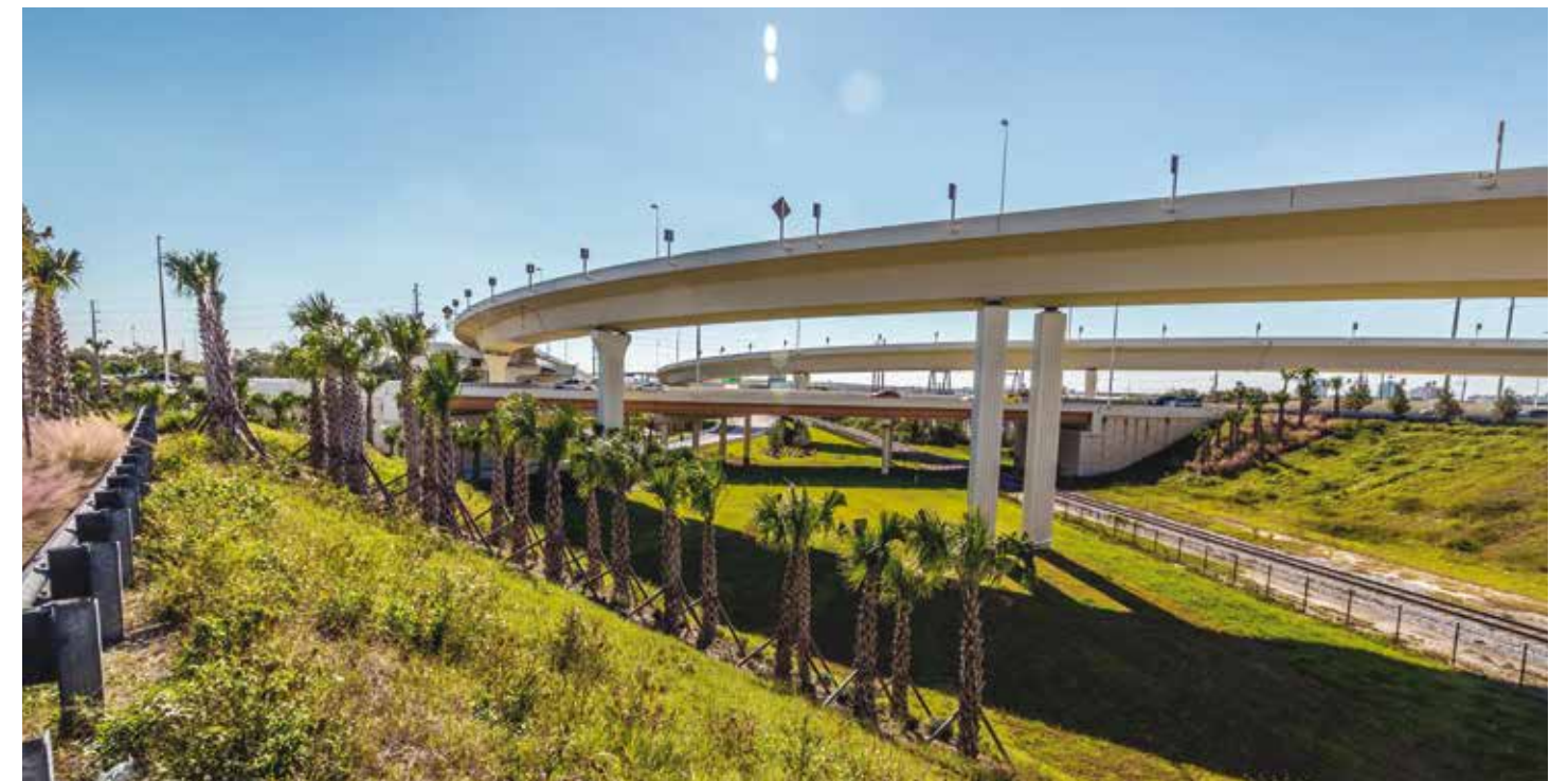
I-4/Selmon Expressway Connector Tampa, Florida Designer, Engineer of Record
