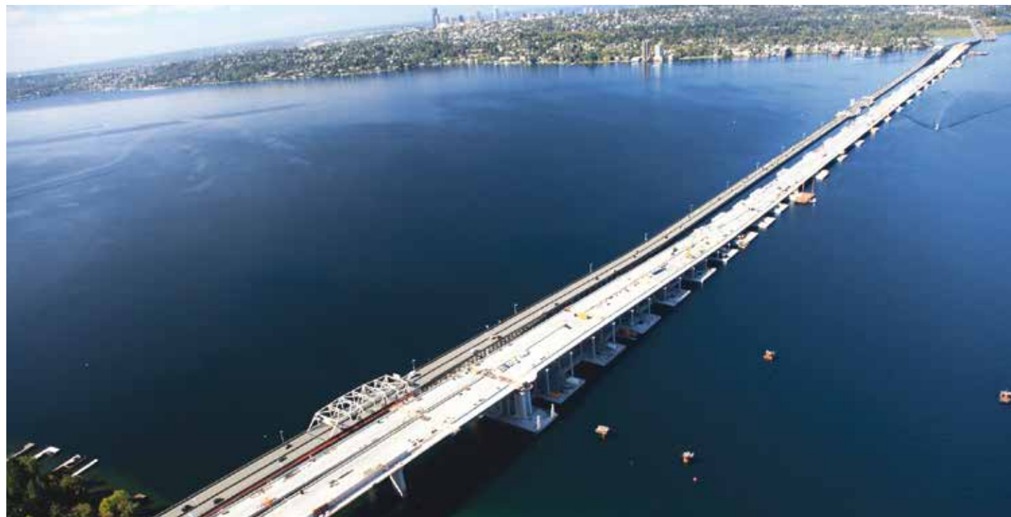
Evergreen Point Floating Bridge (SR 520) Seattle, Washington Program and Project Management Services; Preliminary Engineering; Constuction Oversight
