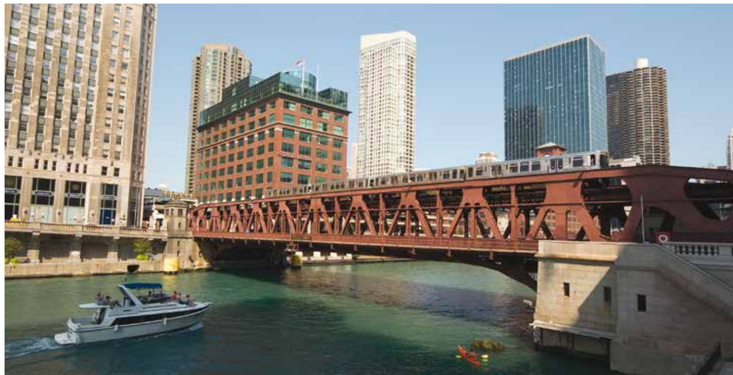
Wells Street Bridge Rehabilitation Chicago, Illinois Construction Engineering
