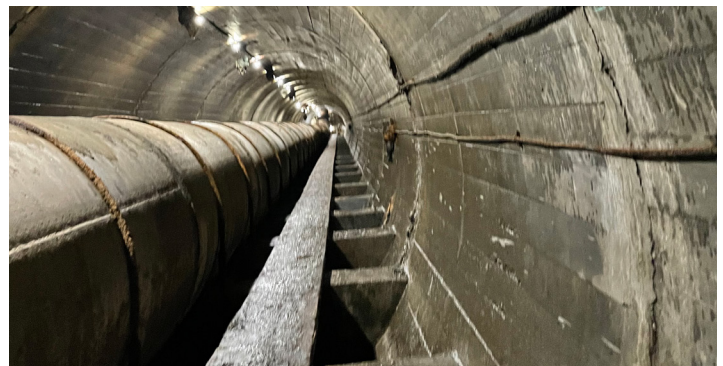
Waterworks Park Transmission Main, MI | WSP designed 4.2 miles of water main which transmits treated, finished drinking water from the Water Works Park Water Treatment Plant (WTP) to the Northeast WTP. Through a progressive design build contract, WSP has assisted the PDB builder and the owner in developing a reduced risk design that repurposes an existing tunnel for a major interstate crossing and developed trenchless solutions for critical crossings in other congested areas.
