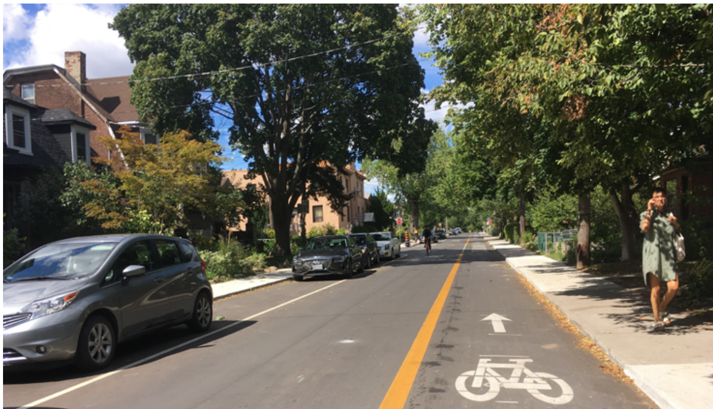
Figure 9: An example of a 7 m wide local street accommodating street parking, two-way bike travel, and one-way vehicle travel.
