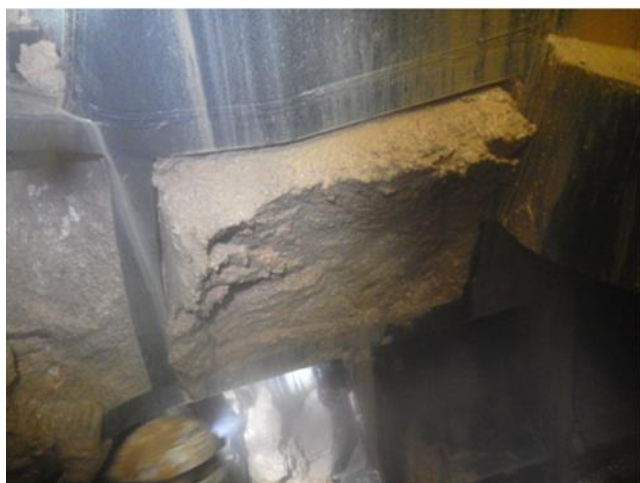
Figure 4. ‘Clayey cdg’ being extruded through an opening in the cutterhead
