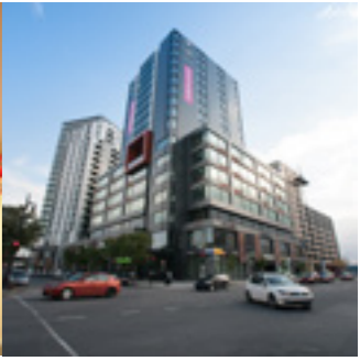
Construction Management District Griffintown – Block 10 Page 49
